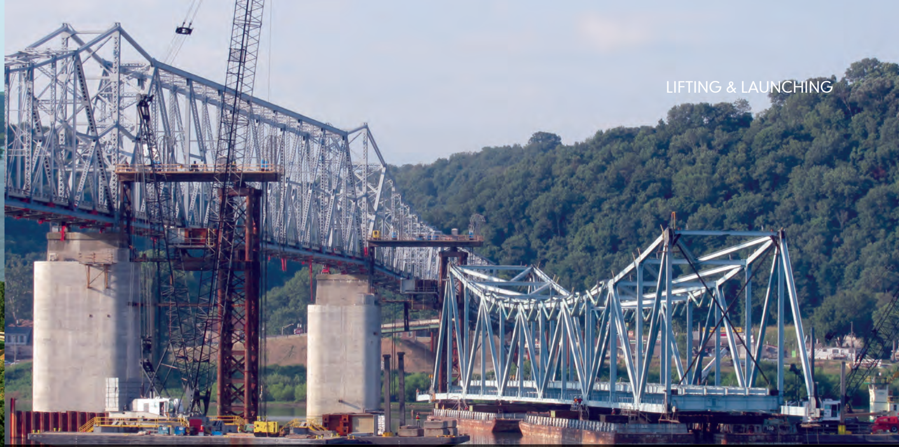
Above: The first major operation under way. Left: The new span on top of the temporary piers
